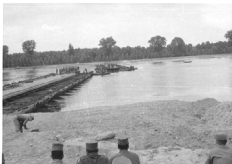
Crossing the Rhine River near Oppenheim, Germany with a Class 60 floating bridge, June 1960.
