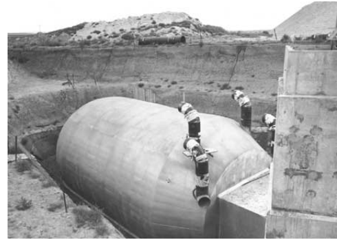
Underground Launch Control Center (LCC) under construction
